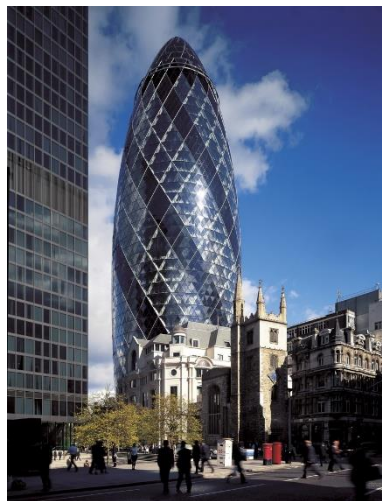
Figura 01 – Torre 30 St. Mary – Norman Foster
